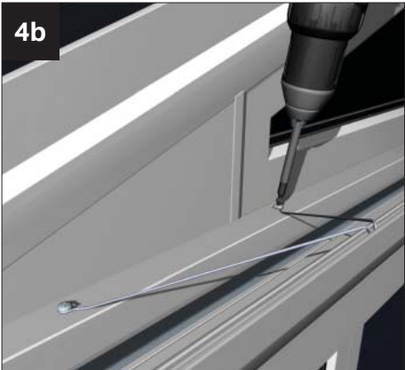
4b Fix wire ties at an angle as shown, ensure the Cornice is parallel to the frames/roof line.
